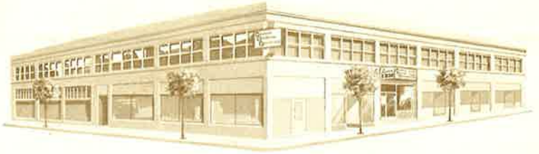
ADMINISTRATION SECRETARIAL SCIENCE BUILDING
